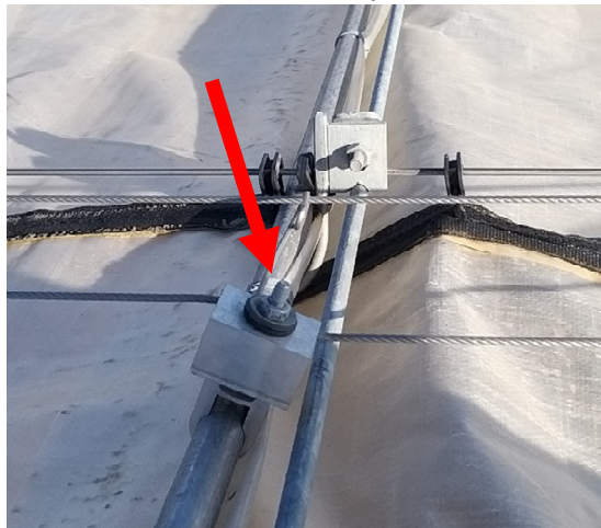
Tube carrier rotates when the leading edge has overtravelled causing cable tension dramatically increase
